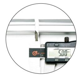
Reserve 5mm of space in between sections of channel to allow for contraction and expansion.
